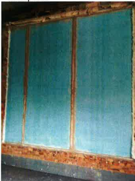
Exposed face before the test
