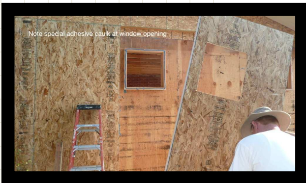
Figure 9. Window Box with Retrofit Panel Courtesy Zero-EnergyPlans.com
