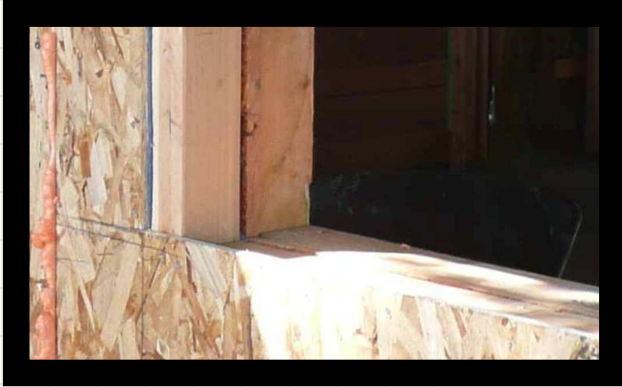
Figure 8. Retrofit Panel Routed for Window Box Courtesy Zero-EnergyPlans.com
