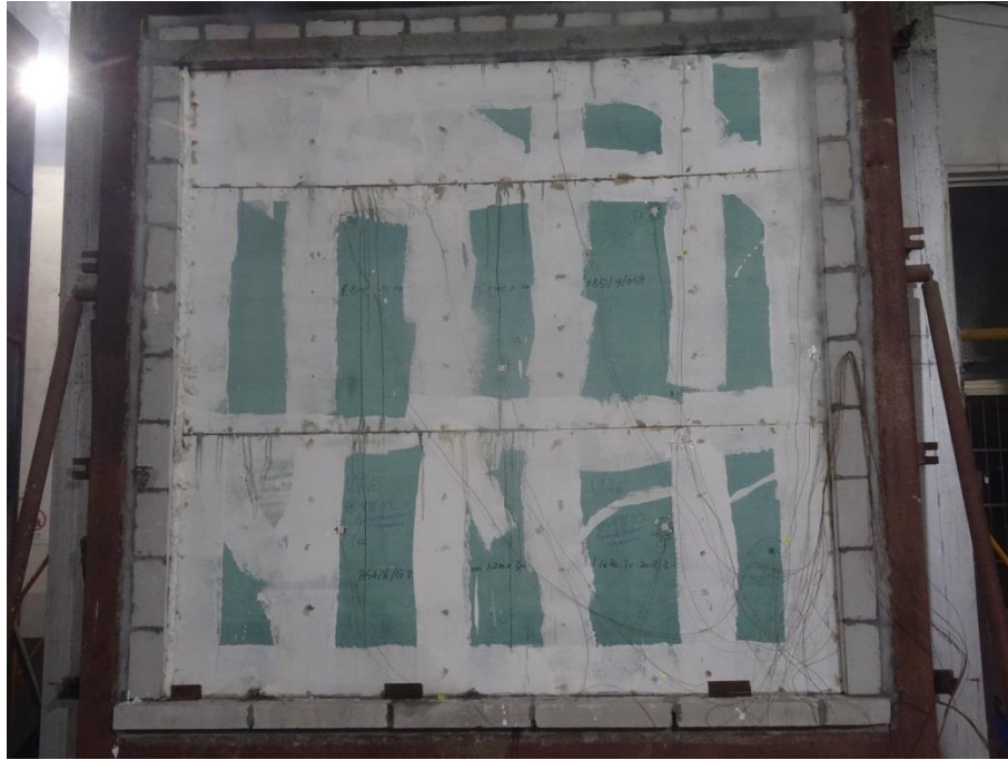
Photo No. 3 Unexposed Side after 30 Minutes
