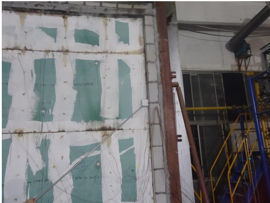
Photo No. 4 Unexposed Side after 90 Minutes
